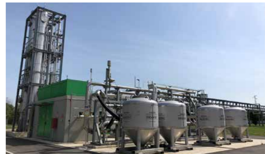
Biomethane production facility at the Bottrighe plant
