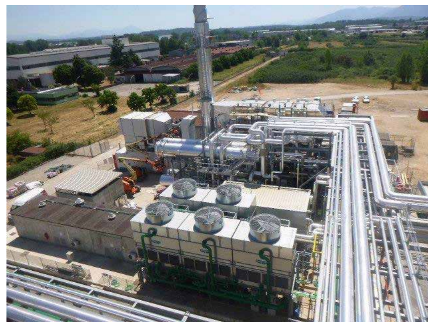
Trigeneration facility at the Patrica plant
