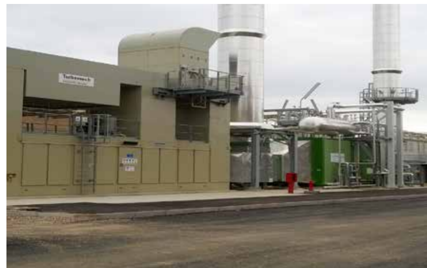
Cogeneration facility at the Bottrighe plant
